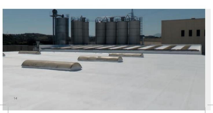
THE STANDOUT CHARACTERISTIC OF THIS LINE IS THE INNOVATIVE CHOICE OF A RESIN CONTAINING A POLYMER WITH A PARTICULAR MOLECULAR STRUCTURE (CORE-SHELL): AN EXTERNAL SHELL WHICH GIVES THE POLYMER STRENGTH, PLUS AN INNER CORE WITH THE PERFORMANCE CHARACTERISTICS OF THE RESIN. THE CORE-SHELL STRUCTURE ENSURES LONGER DURATION WITHOUT ANY DETERIORATION IN PERFORMANCE.
